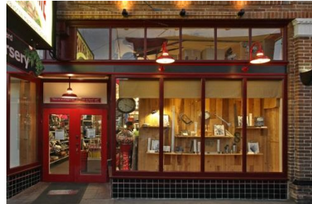
This picture shows an example of the use of borders and offset to denote a change in materials.
