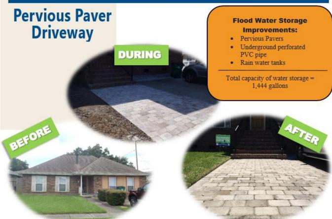
Above: Progression photos of Home #1; the original walkway to the house was torn up to install a pervious paver driveway, which lays on a bed of crushed limestone.
