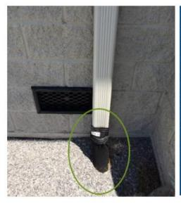
Left: One of two new downspouts installed into the ground. Water flows into a perforated PVC pipe, buried underneath a gravel trench (seen in picture to the right). The pipe disperses water throughout the ground. When the pipe gets too full, the water is directed underground toward the street to drain.
