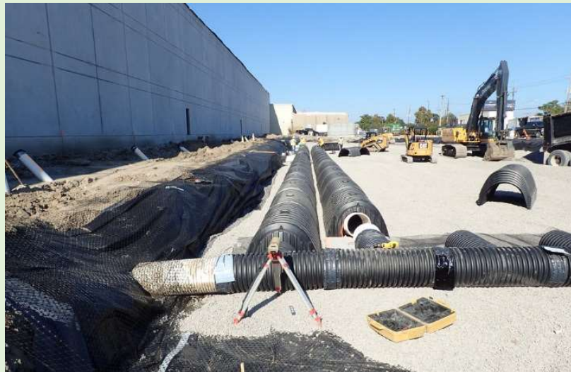
Figure 17a. (Left) Parking lot island retention area at Zuppardo's Market. (Right) Installation of subsurface detention infrastructure at Republic National Distributing. (Credit: Richard Gillian)
