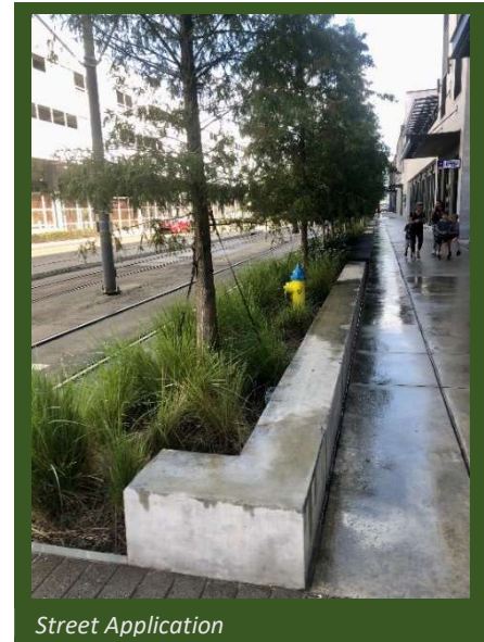
Street Application Figure 15. Street Bioretention in Tampa, FL (Credit: Richard Gillen)
