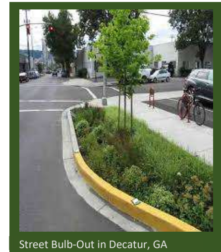
Street Bulb-Out in Decatur, GA Figure 16. Street Bulb-Out with Bioretention (Source: City of Decatur)
